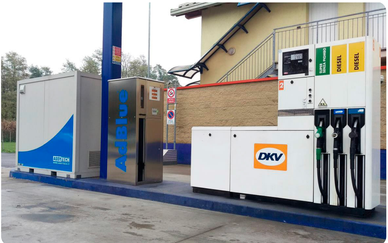
Refueling station with AT30/U dispenser
